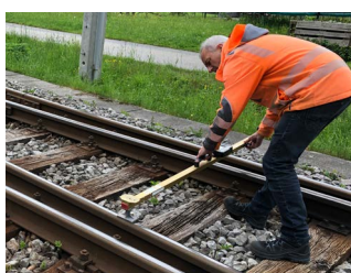
Taking measurements on a switch
