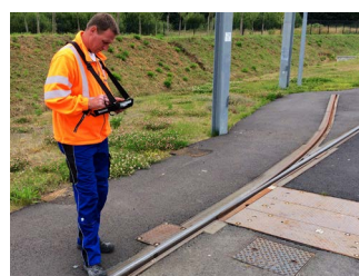
Visual inspection of switch
